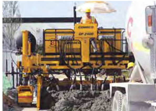
Stringless systems are plug and play technology with the GP-2400's G+ proprietary software and control system.
