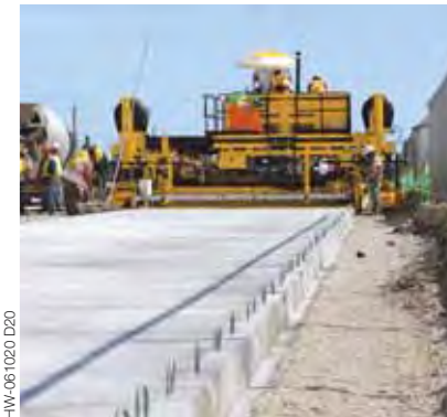
The GP-2400 is capable of slipforming in tight clearance areas.
